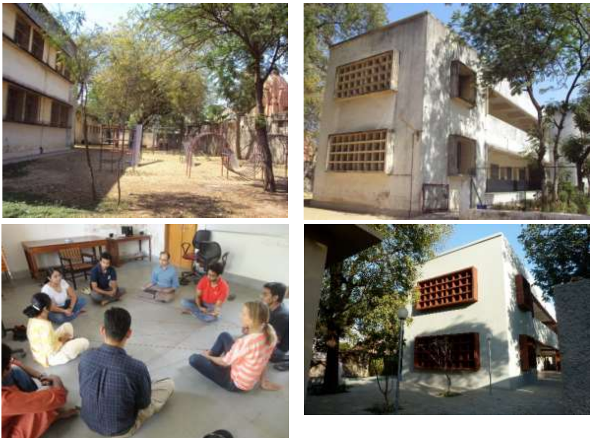
Figure 1: Old physical structure above and renovated structure below
